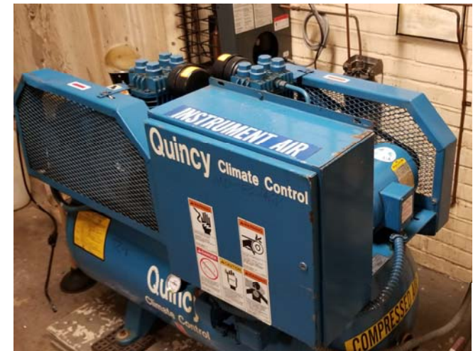
Main mechanical room pneumatic controls
