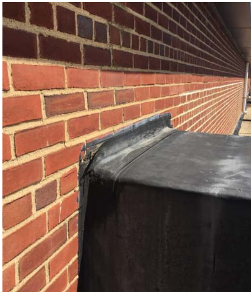
Ductwork penetration with loose flashing
