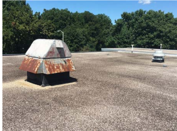
Rusting mechanical equipment on roof
