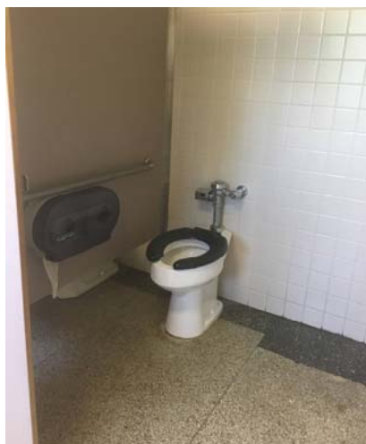
ADA stall dimensions are slightly off and required grab bars not provided
