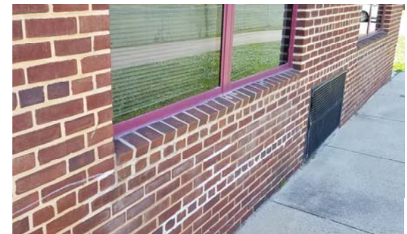
Header brick window sills
