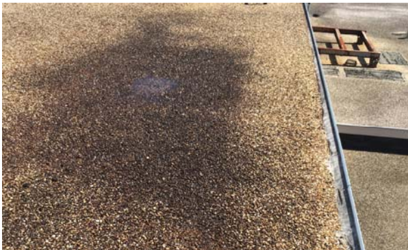
Area of standing water at cafeteria roof
