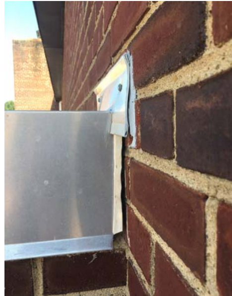
Voids in metal/sealant at coping
