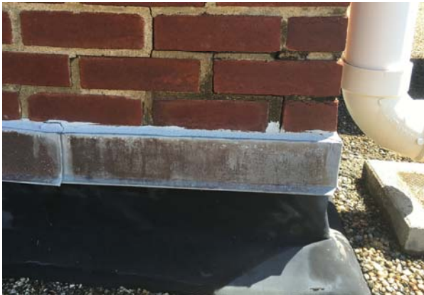
Cracking mortar joints & deteriorating sealant
