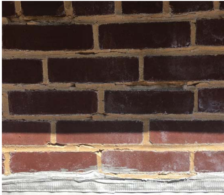
Area of 1952 building needs repointing above roofline
