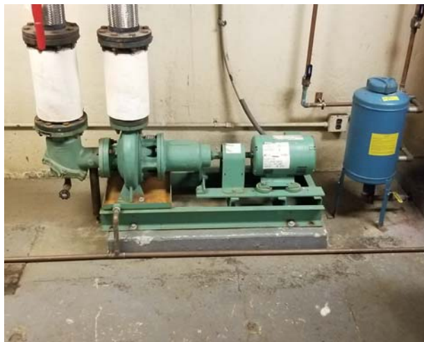
Main mechanical room pumps
