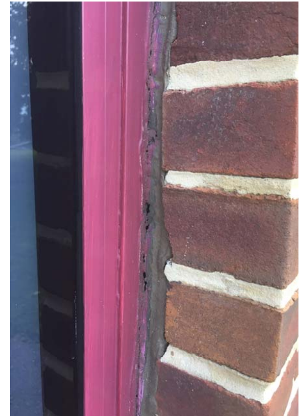
Deteriorating sealant at exterior frame
