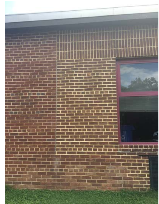
Original 1952 construction with brick infill at old window openings & modified windows
