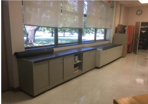
Typical classroom unit ventilator
