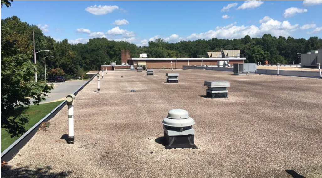
Overview of built-up asphalt roof at original construction south wing
