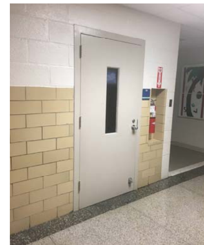
Nearly all of the existing door hardware is non-ADA compliant
